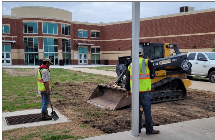
Removing the invasive grass and 2 inches of dirt. Photo by Jaime Flores.
